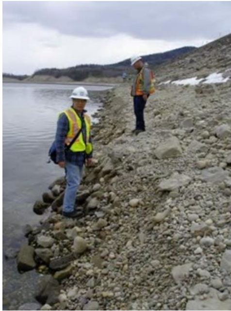
Figure 2 – Riprap at WAC Bennett Dam
