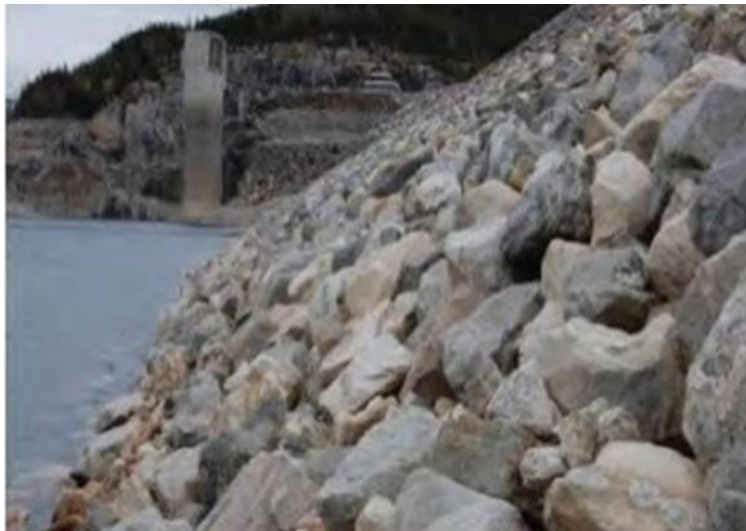
Figure 3 – Riprap at Mica Dam
